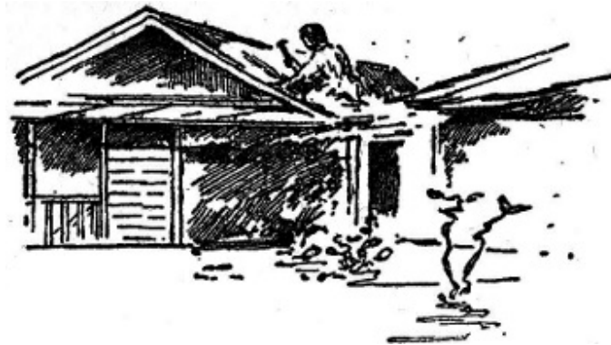
MA MENDING THE ROOF ON SUNDAY.
